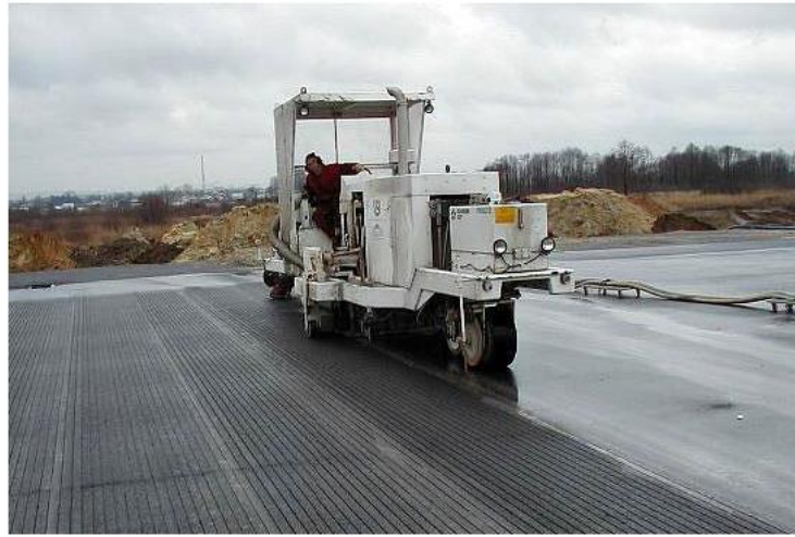
Figure A6-5. Grooving with saws
