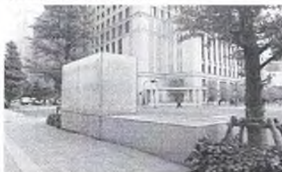
Ventilation / Fire Exhaust
